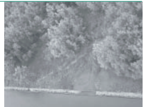
These photos illustrate the longitudinal dikes that were constructed in the late 19 th and early 20 th centuries along the banks of the main channel of the estuary north of the City of Hudson. In many areas such as along the west shore of Schodack Island (above and below right) the trees are growing on dredge spoil deposited in the shallows behind the dikes.
