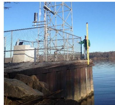
Water Level Station
